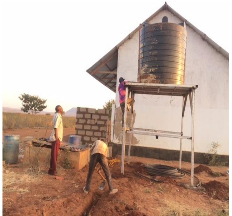
Pumping line installation and storage tank settings
