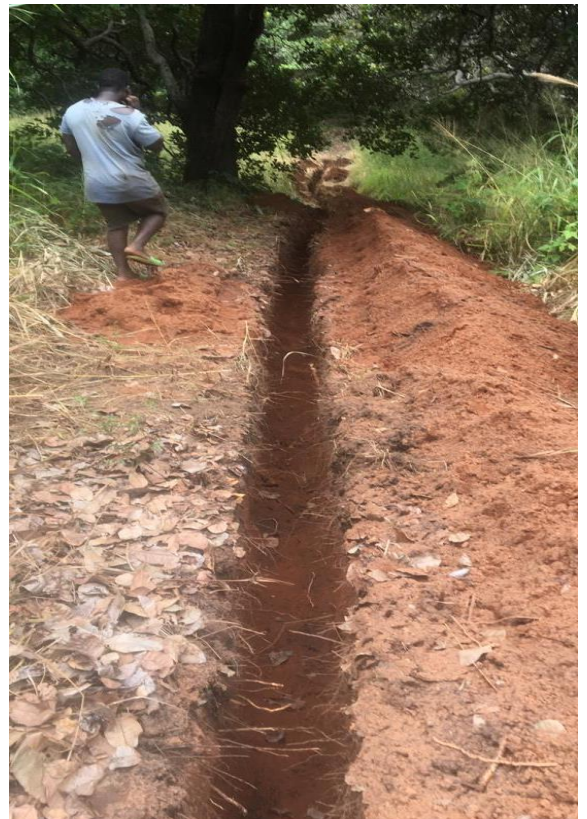
Trench excavation for water pipes installation
