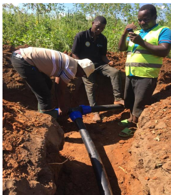
Pipe fixing & junction establishment
