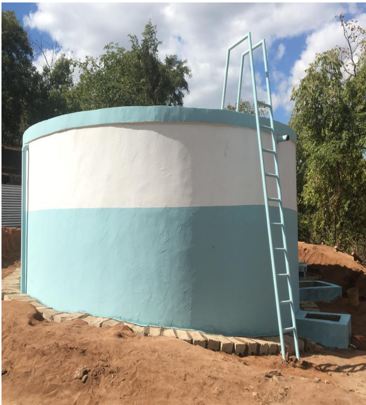
100m 3 storage tank constructed (Msokosela)
